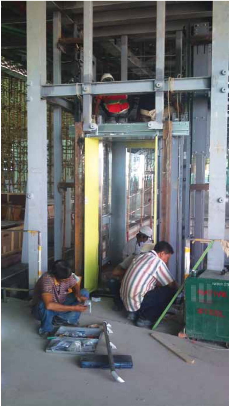
Installing Mitsubishi Elevators at Nay Pyi Taw International Airport
